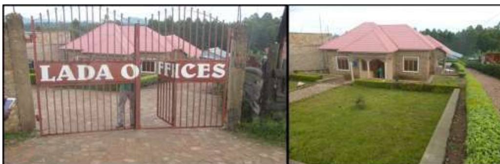
Figure 2.1: Constructed office block.
